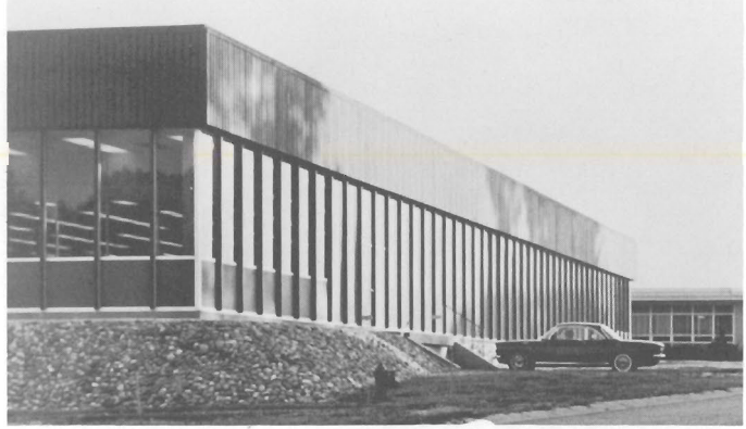
AVONDALE, PENNSYLVANIA—Administrative, marketing, research and engineering groups now occupy this addition at the Avondale Division, completed in May. The 48,000-square-foot building has an aluminum and glass curtain wall topped by vertical steel siding.
